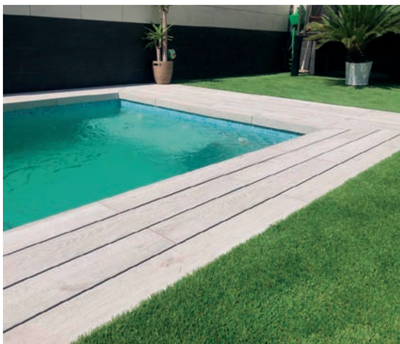
Private house pool · Barcelona · Exadeck natural
